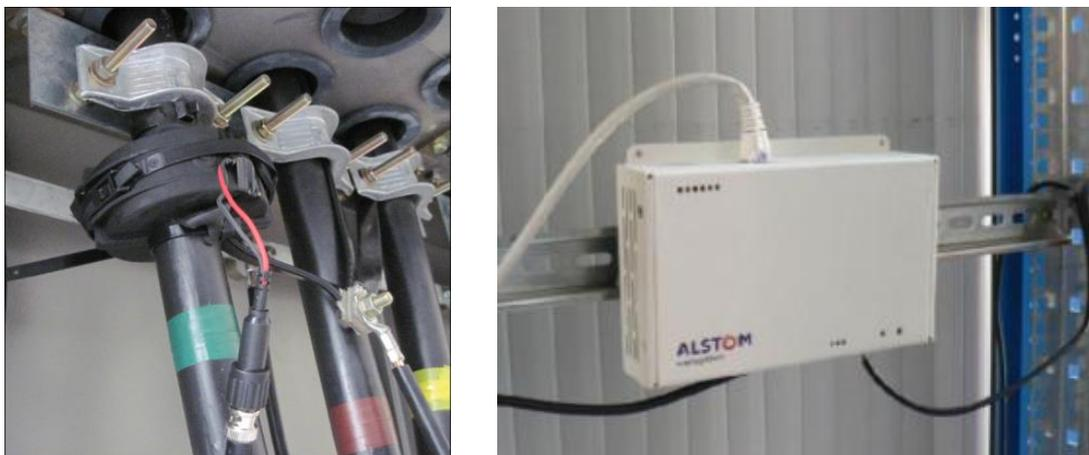
Figure 3 - Inductive coupler on the MV grid and BPL modem at an MV/LV substation
